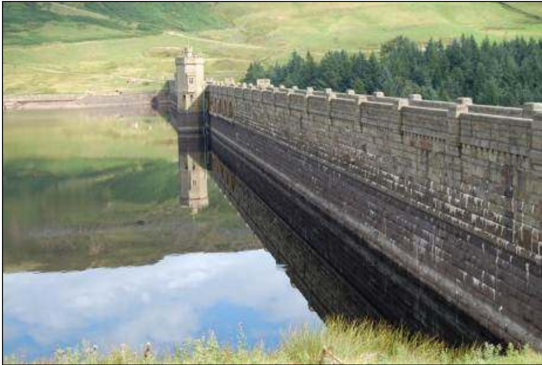
Figure 6: Scar Reservoir Dam Wall 8 th August 2009 (Photograph by author)
