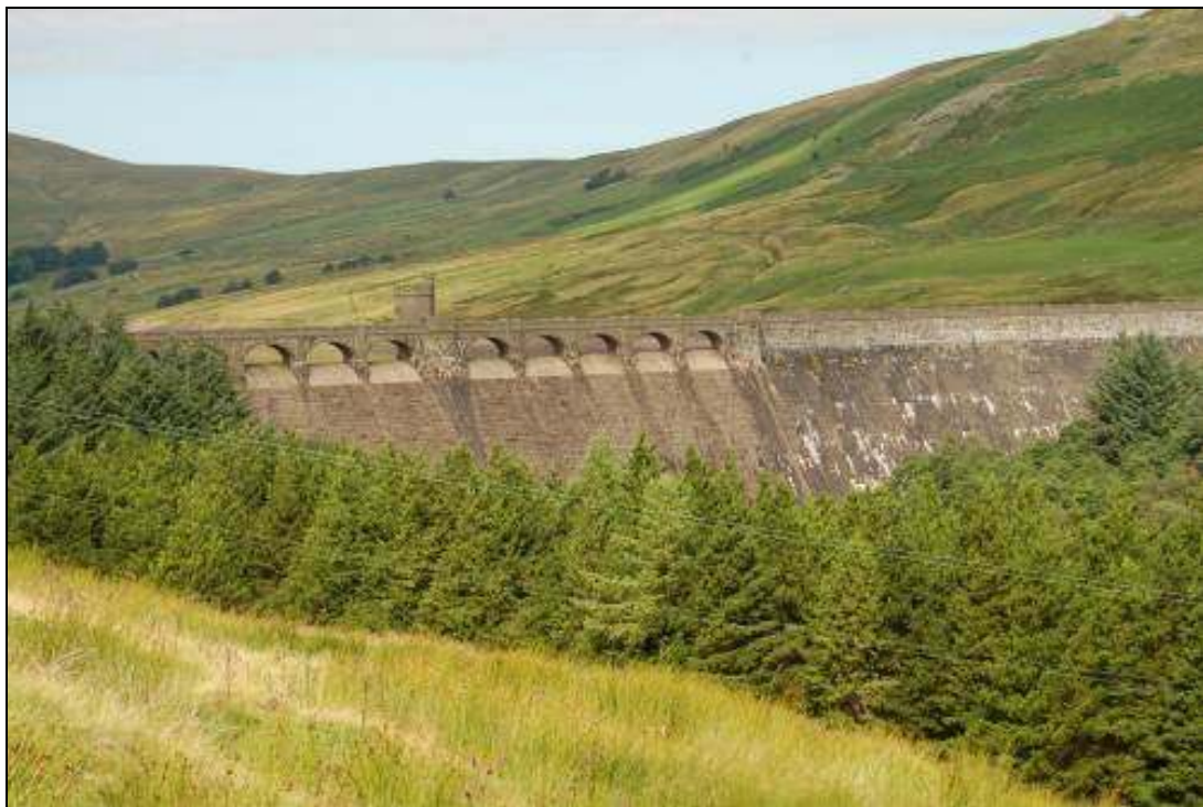
Figure 7: Scar Reservoir Dam Wall.
